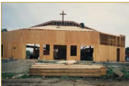
By May of 1988, wood framing was completed, and the church was wrapped in plywood
