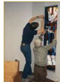
Stain glass windows are installed
